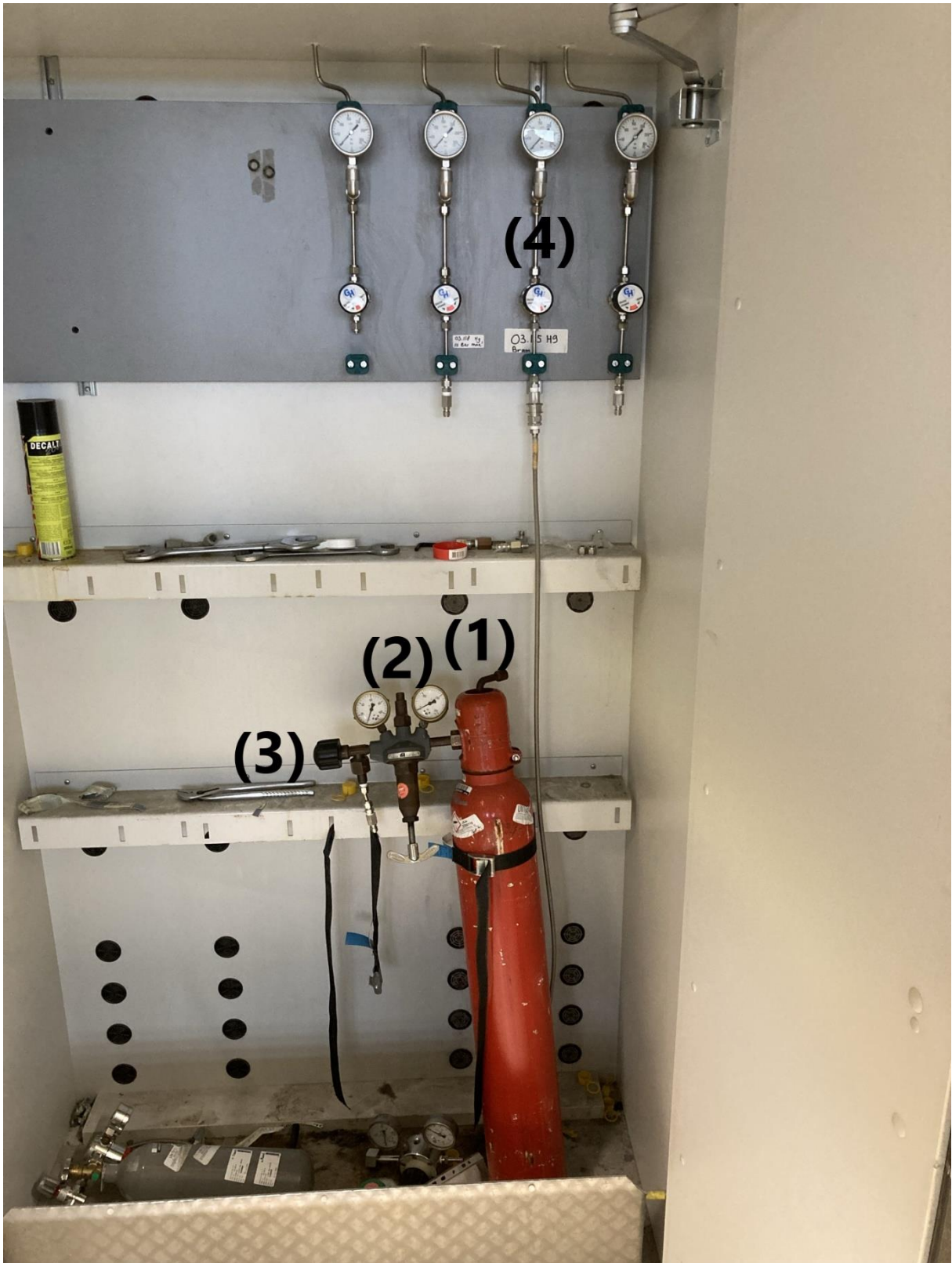
Figure 15: Numbering of valves in the gas cylinder cabinet (HG03-100 GC2)
